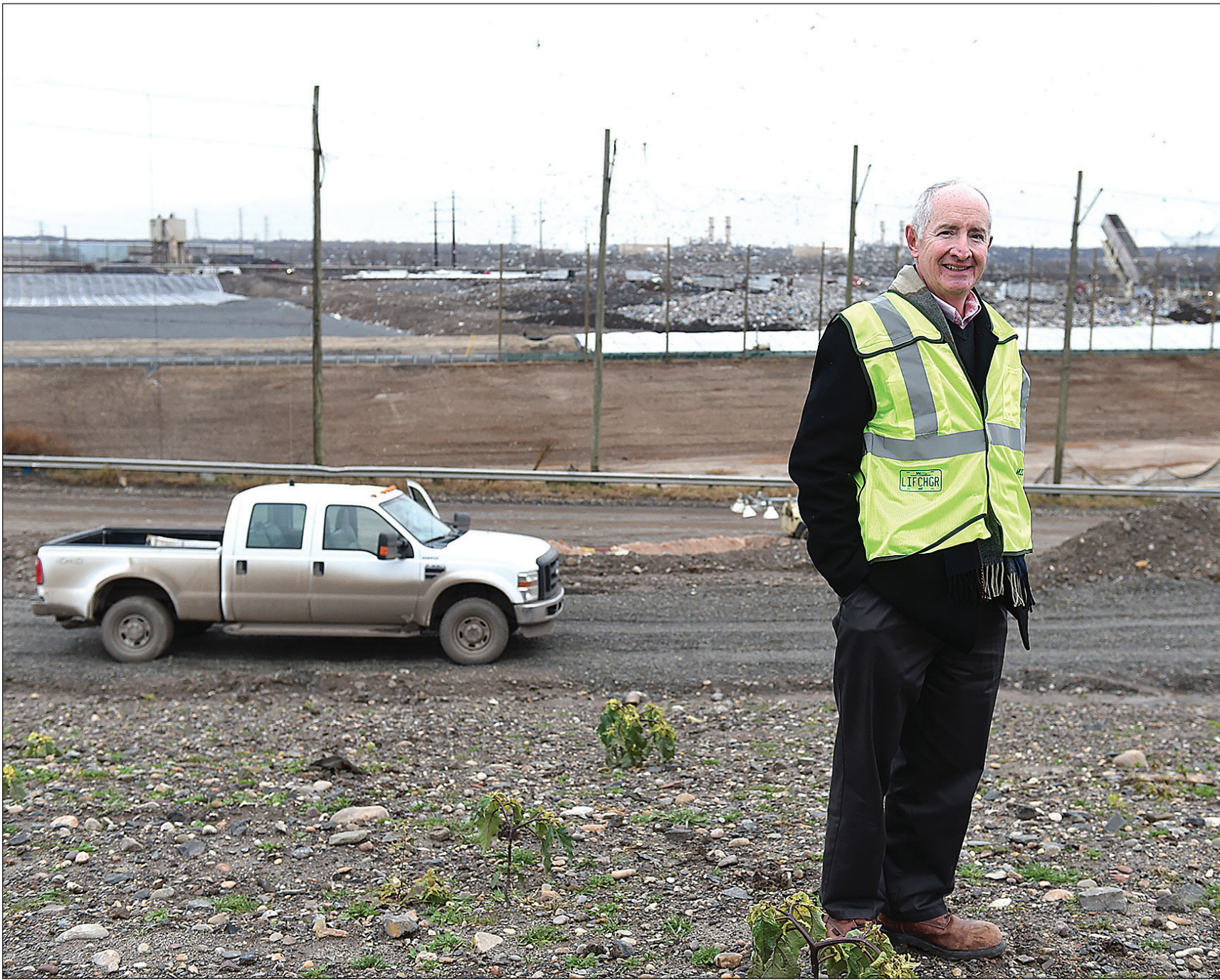
The Waste Management landfill has a variety of pollution control measures, including liner systems, daily soil layering, and water and gas management systems, according to company spokesman John Hambrose.
